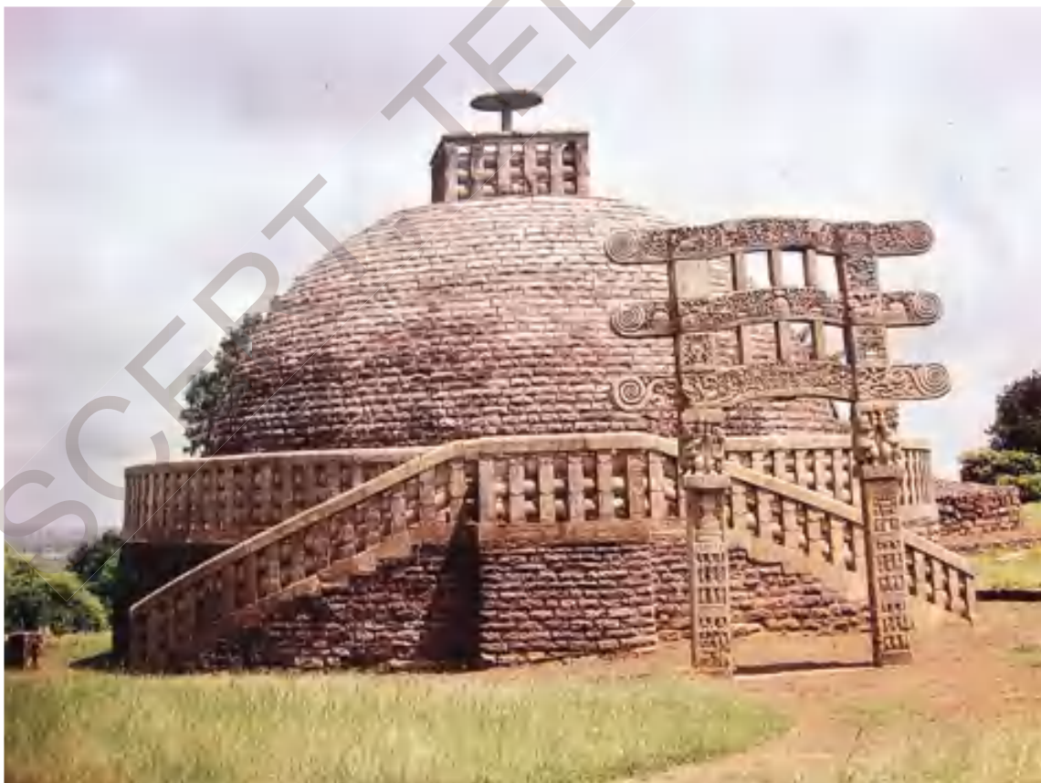
Fig. 20.12: Sanchi stupa in Madhya Pradesh. It is one of the most important stupas built by King Ashoka. Can you identify the hemisphere, the platform, the umbrella and the fence?
